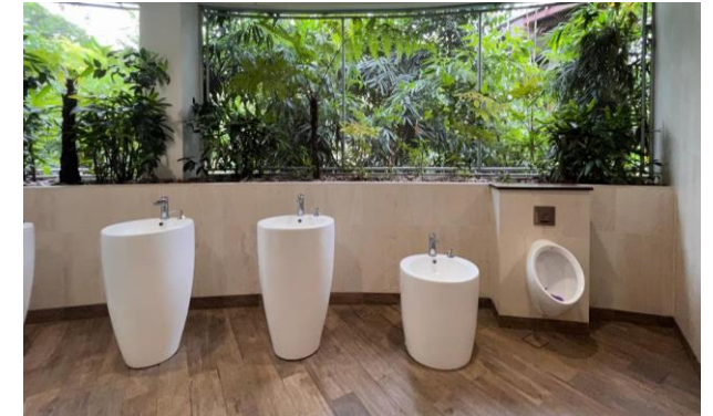
At least one of the wash basins is at a height between 900mm and 1200mm
