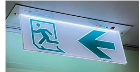
Lighting for emergency exit directional sign
